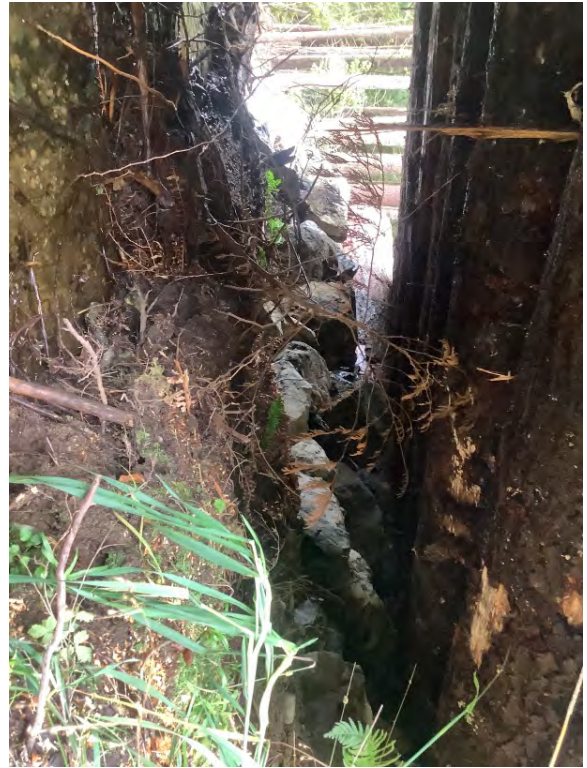
Right Bank Abutment when facing downstream
