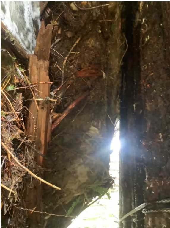
Left Bank Abutment when facing downstream
